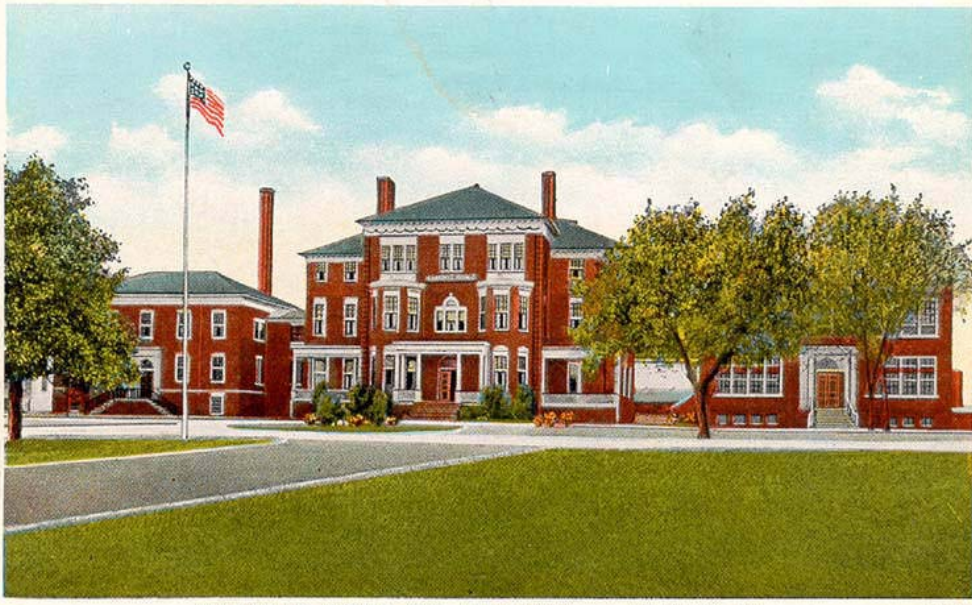
MASONIC HOME OF VIRGINIA — RICHMOND, VA. 4A174
